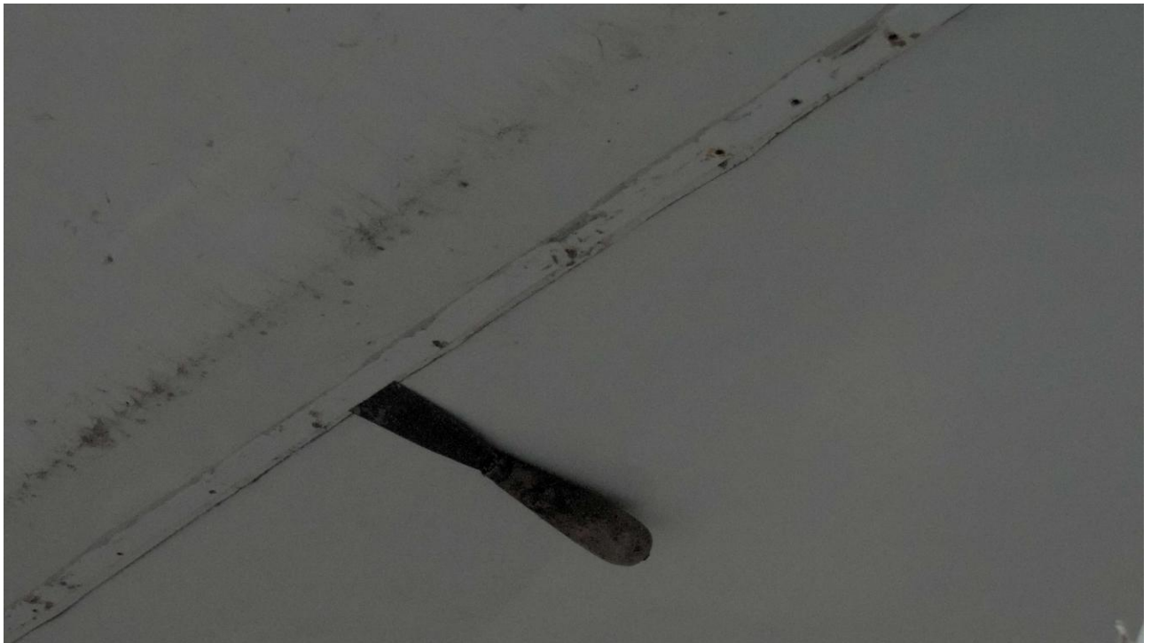
Next is the fibreglass cap on top of the pinbox.
